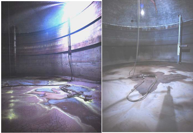
Pictures of 2 SRS Waste Tanks Following Mechanical Cleaning
